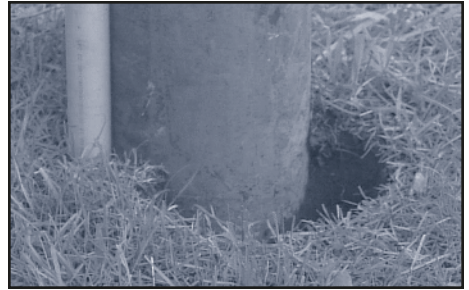
Faulty annular seal.
